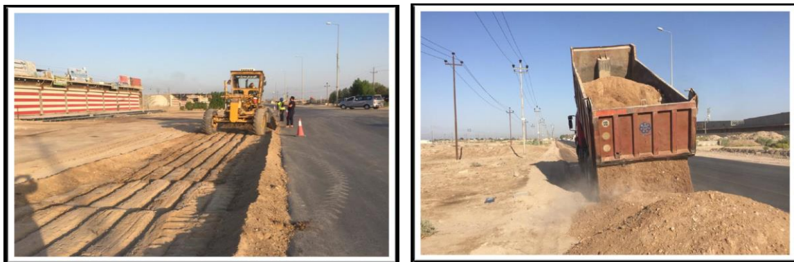
Supply of Street Lights – Al Hartha Area
