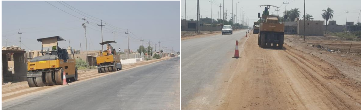
Rehabilitation of Paper Mill Road – Deer Area
